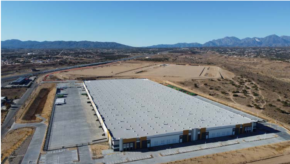
Hesperia Commerce Center One, Building One and Future Building Sites
