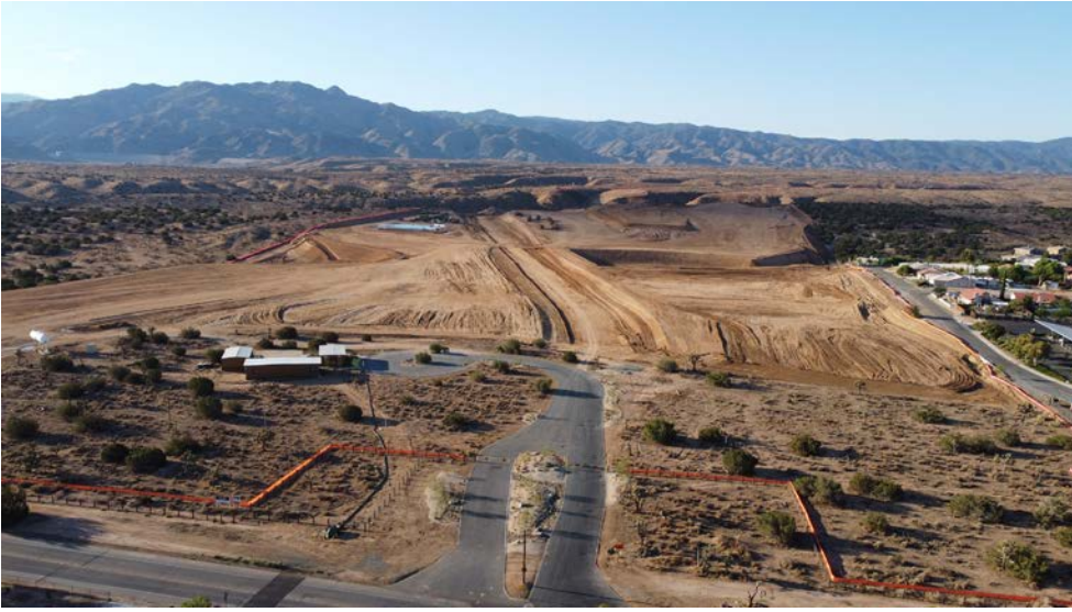
Silverwood Phase One Grading
