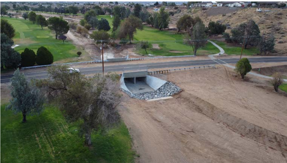
Peach Ave. Drainage Improvement
