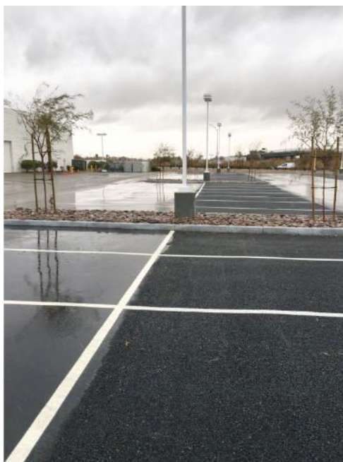
Porous concrete makes up part of a new parking lot in Victorville at Valley Hi Toyota (darker pavement)
